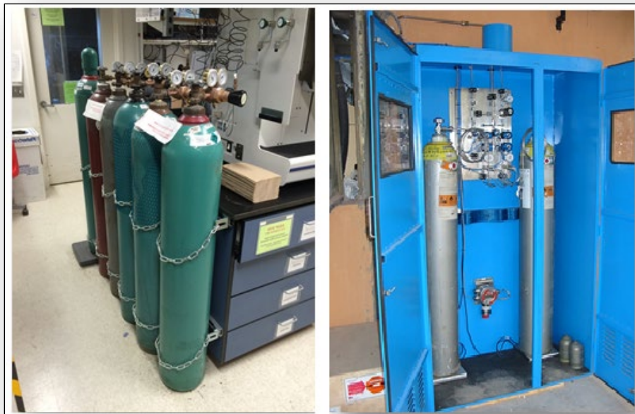
Figure 3.15: Gas Cylinder Storage
