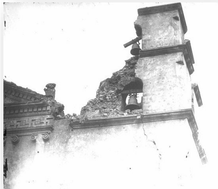
Crumbled bell tower of the Santa Barbara Mission after the 1925 earthquake. Earthquake Engineering Research Center at the UC Berkeley.
